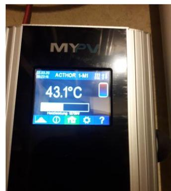
The AC•THOR makes electric heat generators "PV-ready" by linear power control.
