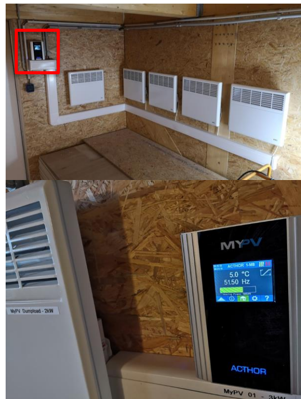
Figure 3 and 4: AC•THORs for electric space heating
